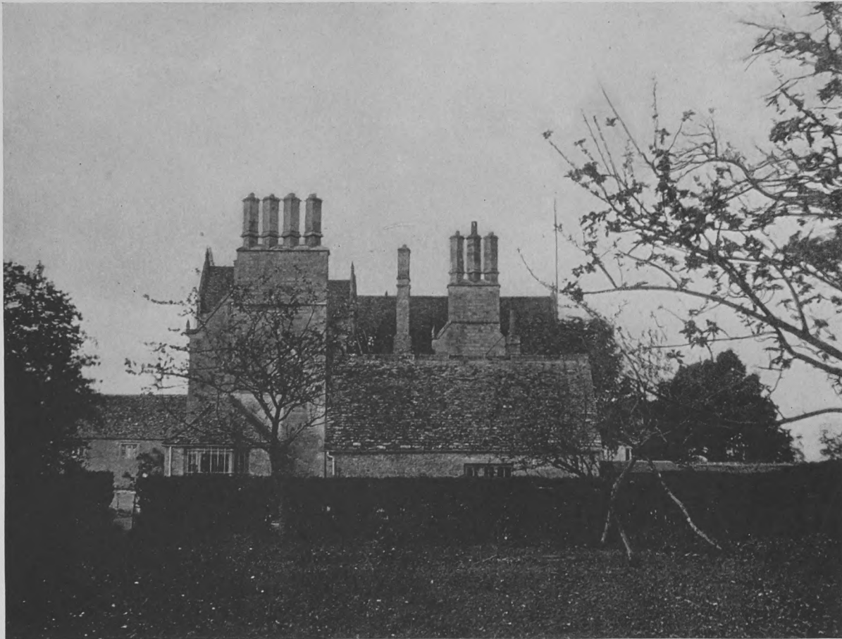
CHIMNEYS AT REAR OF WATER EATON MANOR IN OXFORDSHIRE
